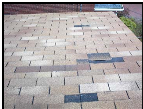
Missing and/or damaged shingles at the rear slope
