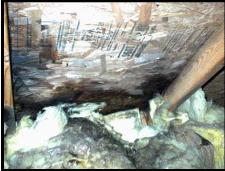
Leakage at skylight as viewed from the attic space.
