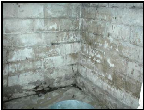
Moisture penetration at the left front corner area of the basement
